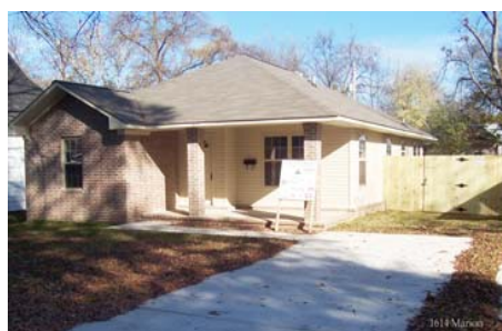
Our energy efficient homes are 1,300 square feet and have three bedrooms, two baths, high efficiency appliances, water and lighting features. Houses are $99,750 with subsidies for qualified buyers up to $20,000.
